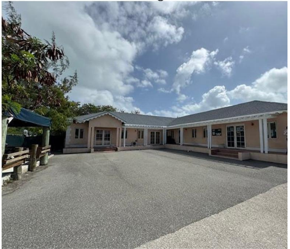
Rear View North Building
