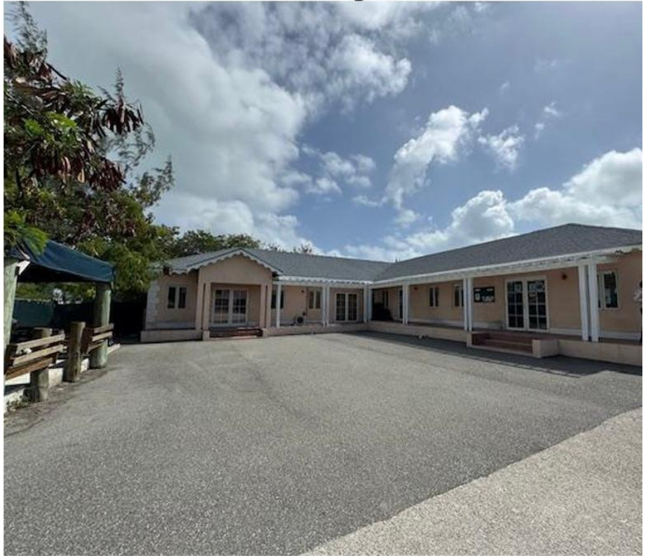
Rear View North Building
