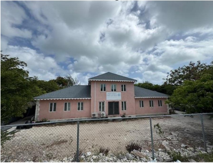
Front View of North Building
